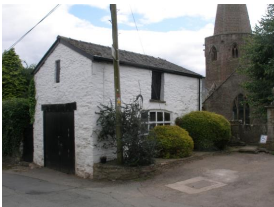
Fig.65 The Coach House to the Post Office. A well preserved simple everyday vernacular building which, like that in Fig.68 are heritage assets contributing to the character of Grosmont.
