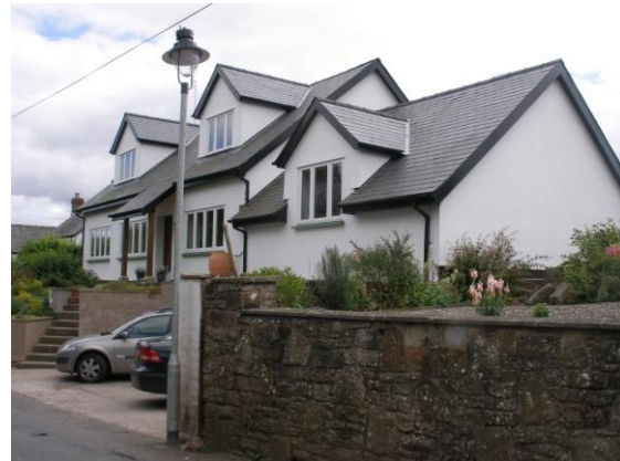
Fig.77 A new wide-fronted house retains the linear building form so characteristic of Grosmont. The subservient wing in the foreground is appropriate in reducing its bulk or repetitive effect. The mullioned windows are also appropriate. Perhaps the dormers could have been slightly less dominant.
