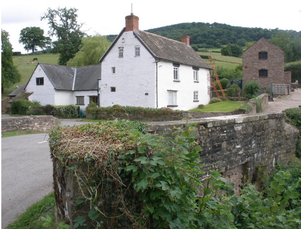
Fig.53 Lower Tresenny Farmhouse. The earliest part dating from the 16 th century is the low wing between the cross wing to the left and the two-storey 'parlour wing' to the right.
