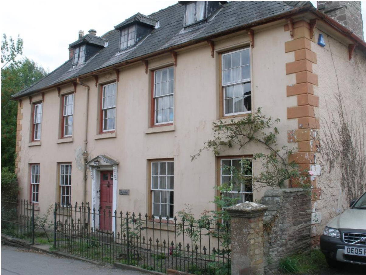
Fig.60 Glyndwr House is a typical renaissance style building, symmetrical, with five bays of sash windows. Pronounced quoins and the steeply pitched roof are typical of the first half of the 18 th century. Here, as in many houses in Grosmont, front boundary railings are an attractive element in the streetscape.
