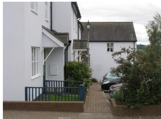
Fig.78 Bevan Court. A courtyard development with appropriate sense of enclosure and massing. The elevations are simple yet have variety. The parking space is well overlooked but not dominant.
