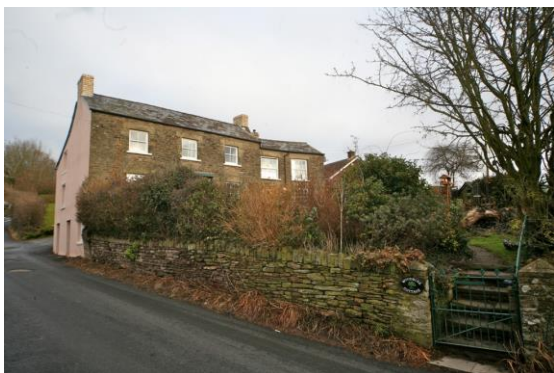
Fig.70 Woodbine Cottage. A mid-19 th century large cottage featuring rubble stone, slate roof and brick end stacks.
