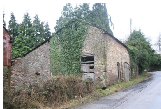
Fig.38 Stone barn opposite Old Tan House
