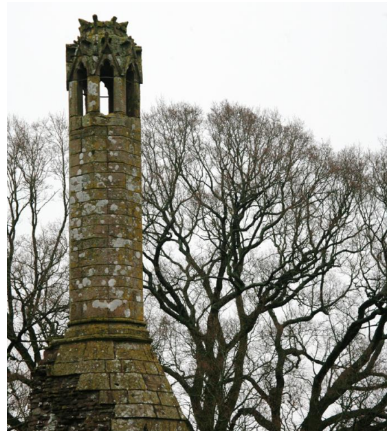
Fig.6 The prominent and distinctive octagonal 14 th century chimney stack, a rare survival at Grosmont Castle
