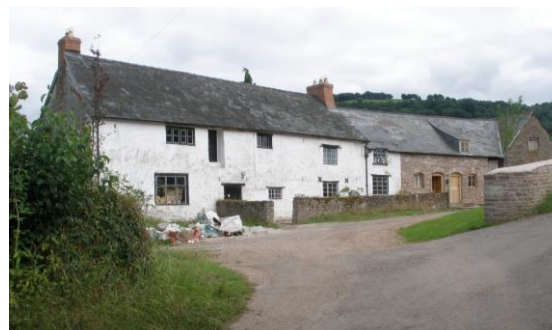
Fig.58 Great Tresenny Farm. The brick stacks mark the extent of the early 17 th century farmhouse with its hall on the left. Subsequent extensions have created a fine range of farm buildings.
