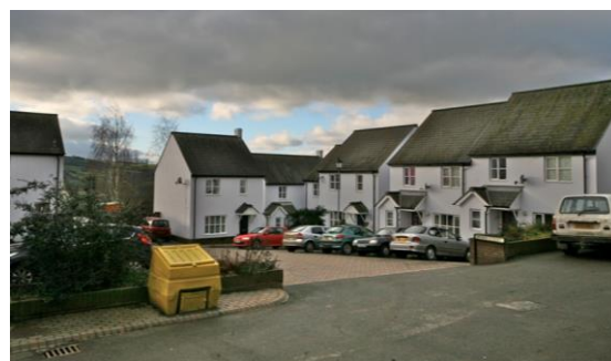
Fig.25 View west with the rendered houses of Bevan Court to the left
