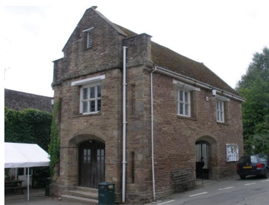
Fig.67 The Town Hall. This was rebuilt in 1831-2 in a hybrid style, recalling 17 th century characteristics, especially with the mullioned and transomed windows. As usual with these buildings, it served as a market hall on the ground floor.
