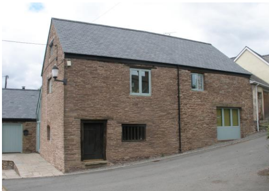
Fig.75 Stable range to Town End Barn is a recent conversion to residential use. Existing openings are utilised, and the simplicity of the original building is retained.
