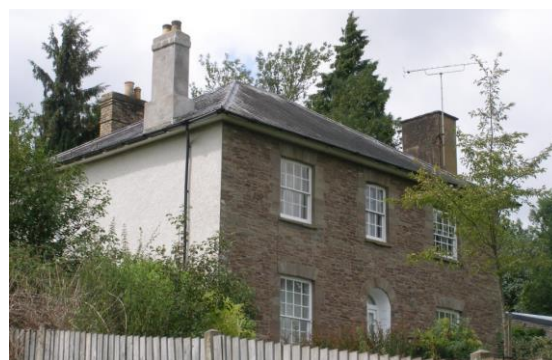
Fig.73 The Old Tan House. Another Regency style house with typical hipped roof, elegant sash windows and semicircular door head.
