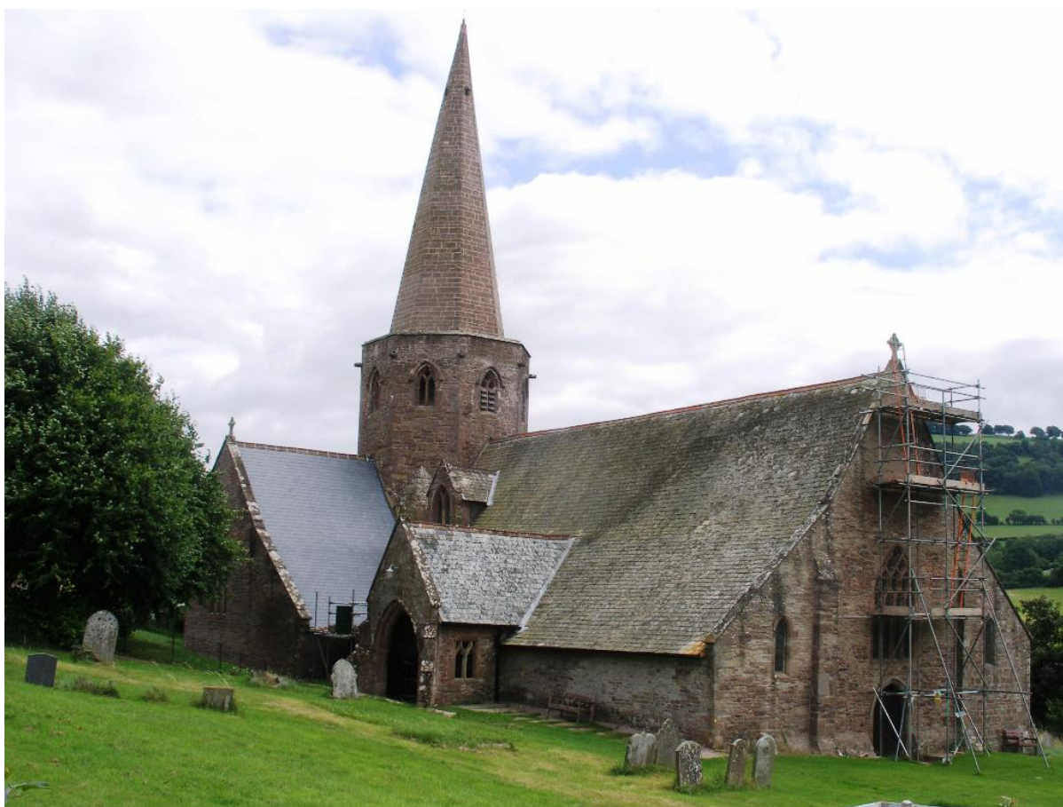
Fig.48 St Nicholas Church from the north-west, showing the barn-like sweep of its nave and transept roof, uninterrupted by clerestory windows. The octagonal tower topped by its spire enhances the significance of this important church
