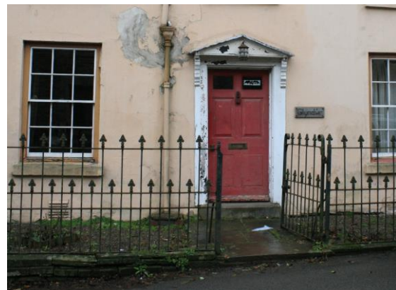
Fig.19 Cast iron railings are a notable surviving feature to some of the grander houses in the conservation area
