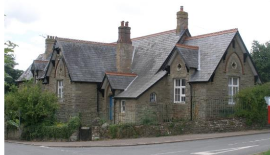
Fig.74 The Old School. The profusion of steeply pitched roofs, tall chimneys and Gothic details such as the quatrefoil vents in the gable ends typify this Victorian Gothic Revival building.
