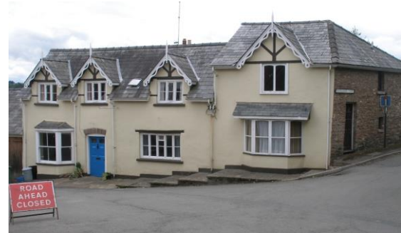
Fig.59 York House was altered and extended (to the right) in the 18 th century. The decorative bargeboards are probably a later feature.
