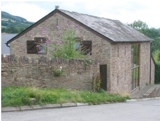
Fig.76 Town Barn. A residential conversion where existing openings, in this case the large cart doorway and the slit vents, have been retained and new windows inserted.
