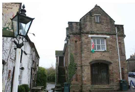
Fig.14 The Town Hall & Angel Public House with narrow lane between the two
