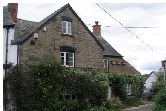
Fig.56 The former Greyhound Inn. The large gable was added somewhat later to this simple wide fronted 17 th century town house.
