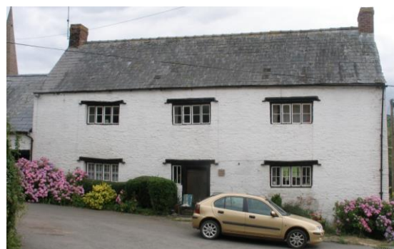
Fig.57 Town Farm House. This remarkably well preserved building of the 17 th century retains its symmetrical façade design of five mullioned windows and central front door. The gable end stacks are a typical feature
