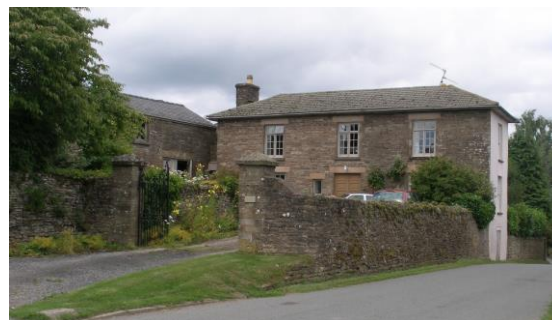
Fig.72 Belgrave House, towards the northern edge of the town, is sited at right angles to the High Street. This broad fronted Regency house has a characteristic low-pitched hipped roof.
