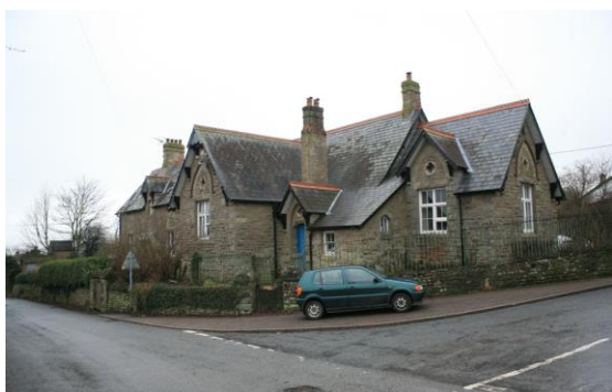
Fig.29 Rock-faced stone used to good effect in the Grade II listed Gothic style school building
