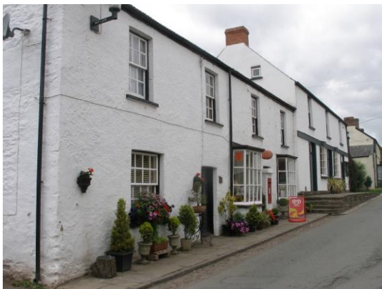
Fig.64 The Post Office, adjoining 'Gentle Jane' steps down the High Street. Its windows are late Georgian in design and the early shopfronts are of particular interest
