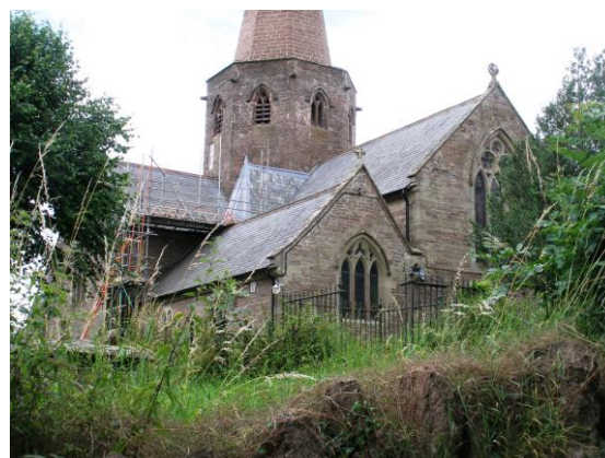
Fig.49 St Nicholas Church from the south-east showing the Victorian rebuilding and restoration of the chancel and chapel
