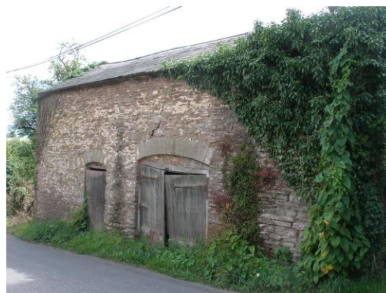
Fig.66 A disused farm building distinguished by well formed voussoirs, stands at the roadside opposite the Old Tan House. Traces of original paintwork can be detected on the rubble walls.
